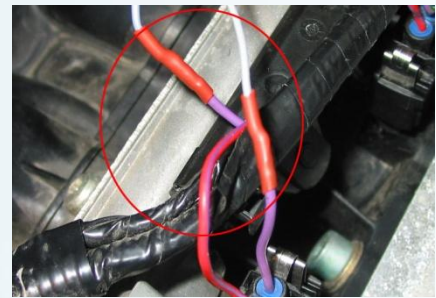
Picture 2f: incorrect wire fitting
